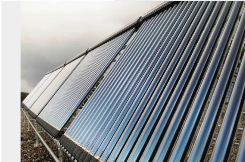
A view of some of the panels which are part of the 15 panel, solar thermal array of vacuum tubes on the roof of the Glens Falls Hospital Renal Dialysis Center on Monday, June 25, 2012 in Glens Falls, NY. A media event was held on Monday to show the installed solar thermal system. The Center uses 200 gallons of heated water per hour for patient treatment, and now has become one of the first in the U.S. to use solar thermal technology for dialysis treatments. (Paul Buckowski / Times Union)
